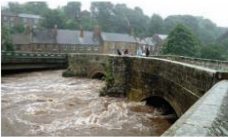
Figure 14: Flooding at Felton on 6 September 2008 (Northumbria County Council, 2008)
